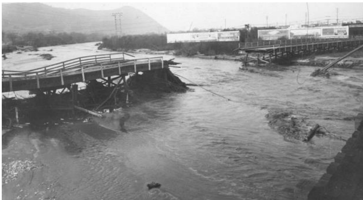
Figure 2-17 Washout of the old trestle bridge at the Glendale-Hyperion viaduct in a photograph dated July 1927. Willow woodlands are visible upstream. Floodwaters have filled the active channel and are close to inundating the floodplain. Los Angeles City Historical Society F-0723. Source: Los Angeles City Archives, Public Works Collection.
