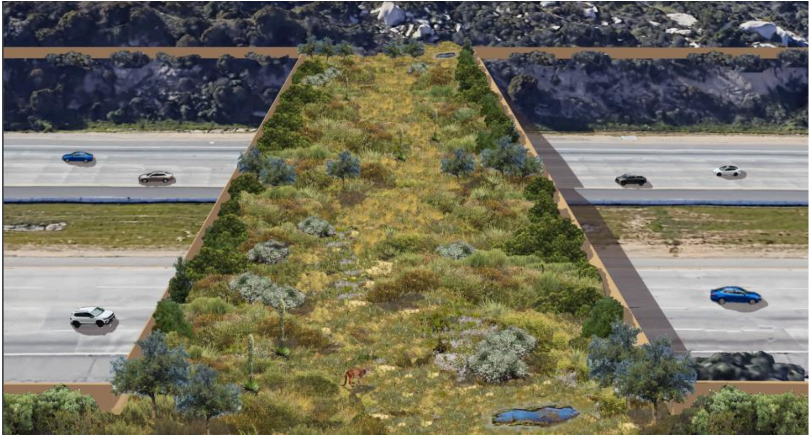
Figure 5: Illustration of Vegetated Wildlife Overcrossing Design Concept (Lance Valley).
